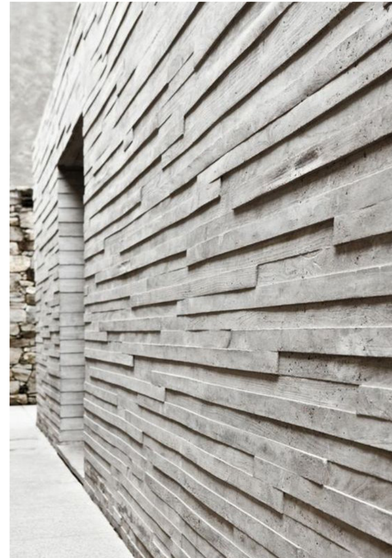
BOARD FORM CONCRET W/ STRONG EDGE DETAIL
