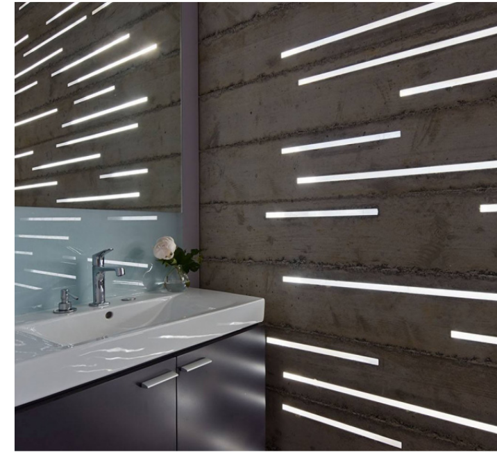
LT-3 STRIP LIGHT INSIDE BUILT-IN CONCRETE FORM
